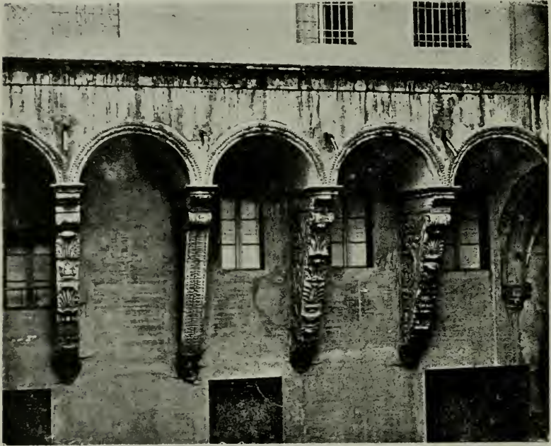
ARCADE ON CORBELS IN CORTILE OF PALAZZO FAVA, BOLOGNA.
